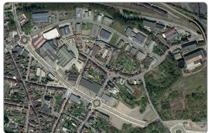
Urban renovation in Seraing (West of Liège, Wallonia). Former colliery site reconverted into commercial and service area. Source : Walloon map – SPW
