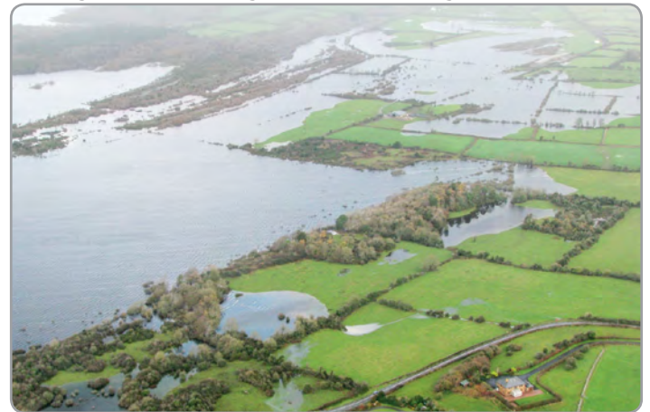
Groundwater flooding in County Galway, Western Ireland, 2016.
